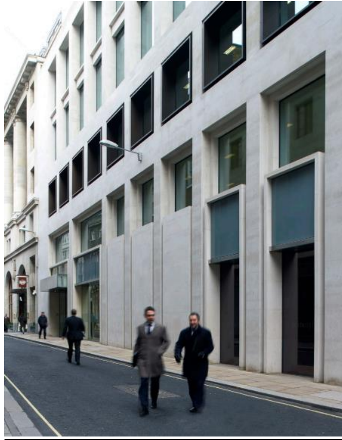
Old Jewry street frontage – west elevation
